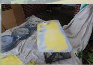
Got a small break in the weather and decided to paint the trunk lid (Boot), the hood (Bonnet), and the outside of the rims that show when on the car.I added a catalysis hardener and some Japan Dryer to the paint and thinned with Acetone. Shot it with 30 PSI at the HVLP gun. While spraying the tack coat, I thought that the paint was coming out a little thick and next time
